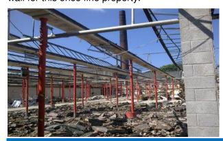
Work on the demolition of the mill commenced during June 2011 with the methodical dismantling of the structure and careful segregation of salvageable materials.
